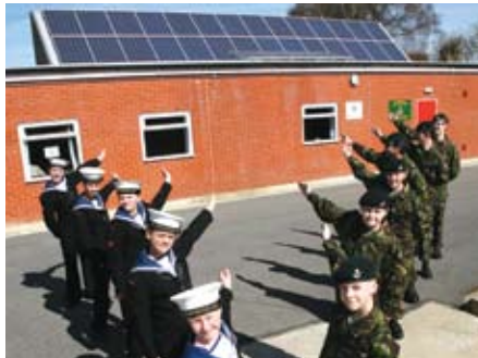
The first Solar PV powered cadet hut in the UK at the Banbury joint Sea and Army Cadet Detachment.
