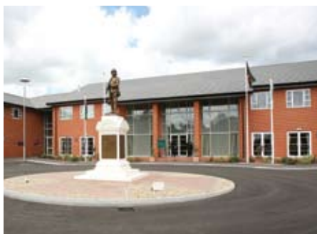
Edward Brooks Barracks, Abingdon.
